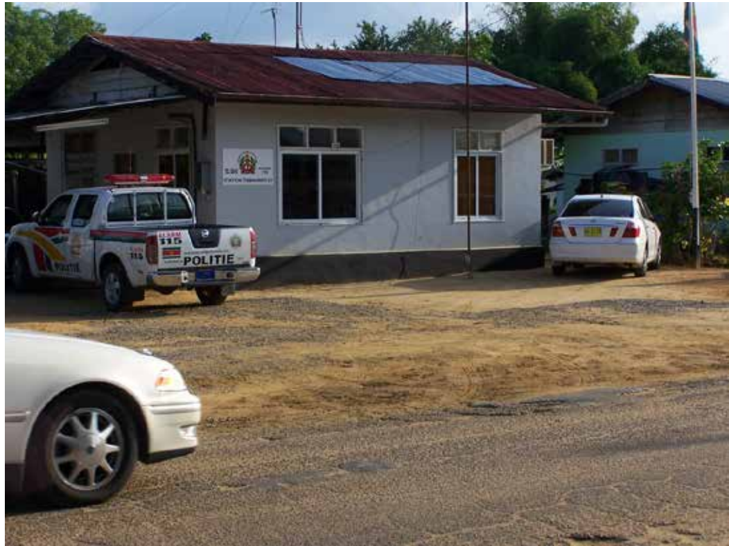
Figure 10-6 Tamanredjo Police Station, Approximately 5m from the East-West Highway
