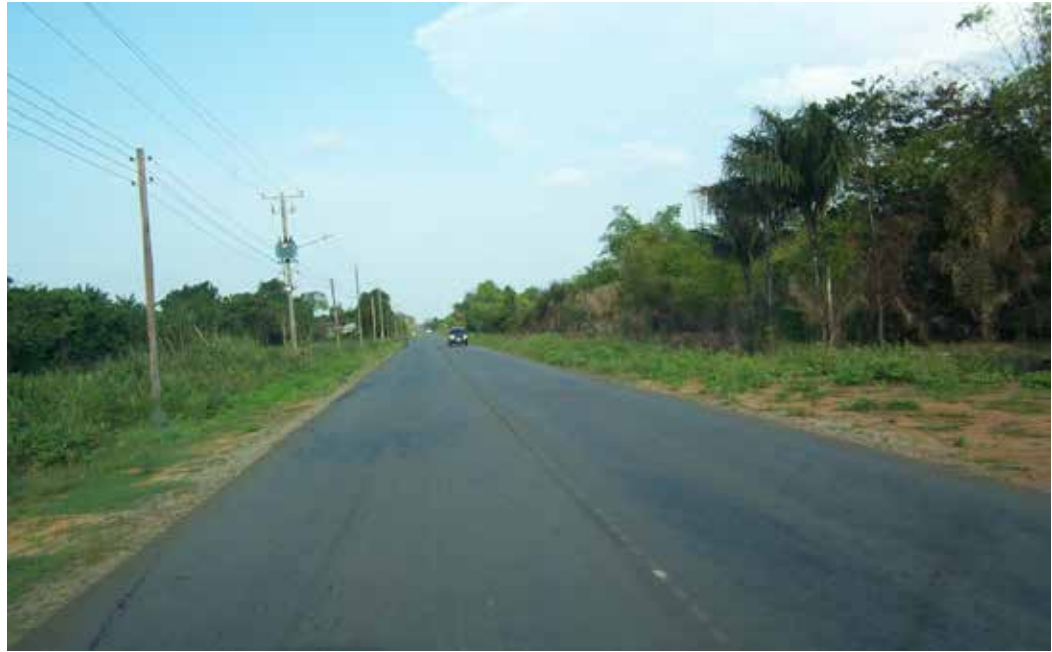
Figure 10-2 The East-West Highway, East of Tamanredjo
