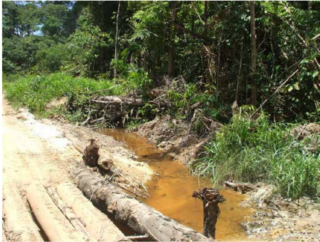
Figure 9-10 Looking Upstream at SW-35 (North Fork A3 Creek - August 2011)
