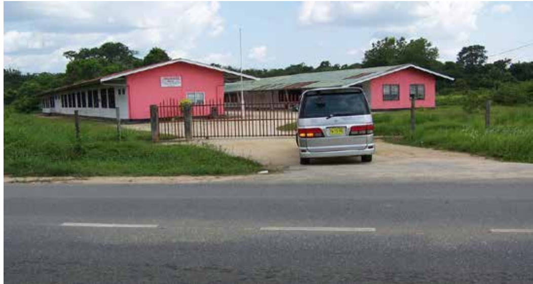
Figure 10-5 Sewrajsing School, East of Bosje Brug, Approximately 20m from the East-West Highway
