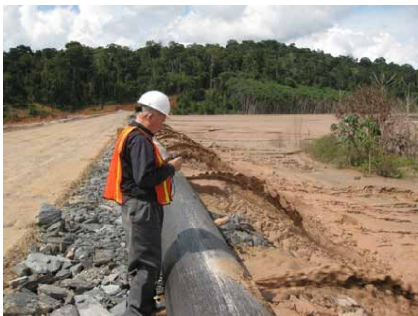
Figure 3-6 Spigotting underway at mine in Guiana Shield
